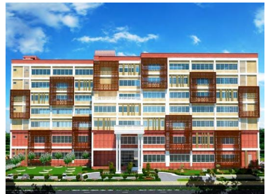
Proposed Redevelopment of Govt. of India Press at Minto Road, New Delhi
