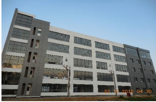
New Administrative Building at NIT Silchar
