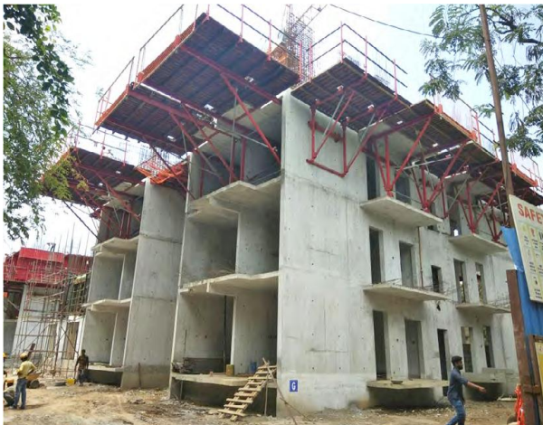
Quarters with Monolithic Construction (New Technology) at Chennai
