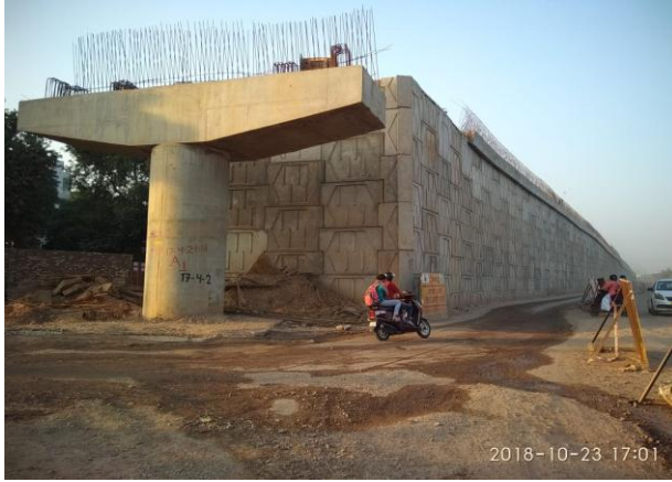
Underpass and Flyover at Mahipalpur, New Delhi
