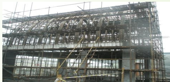
Figure 5 : Bamboo Vault
