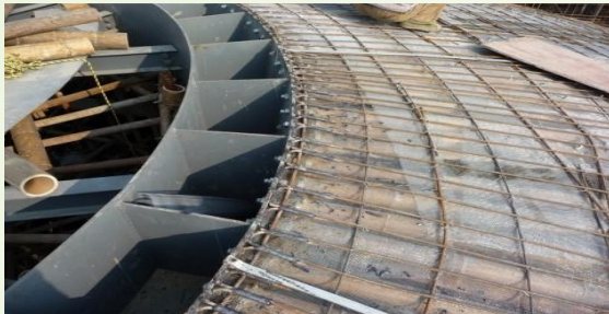
Figure 8 : Wire mesh for ferro-cement layer
