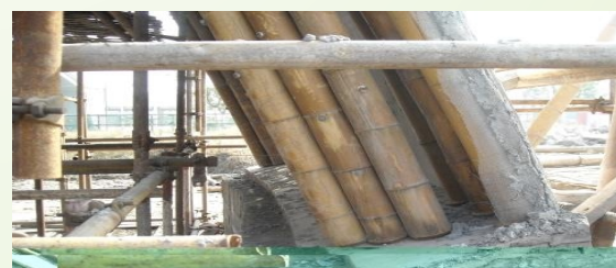
Figure 13 : Mock up for bamboo main beams
