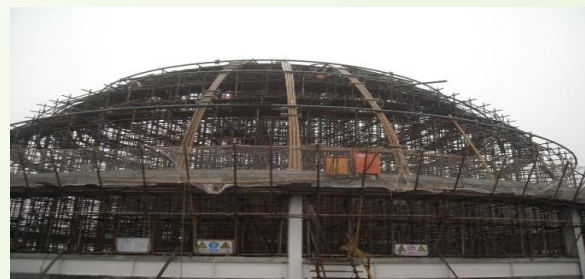
Figure 7: Bamboo structure
