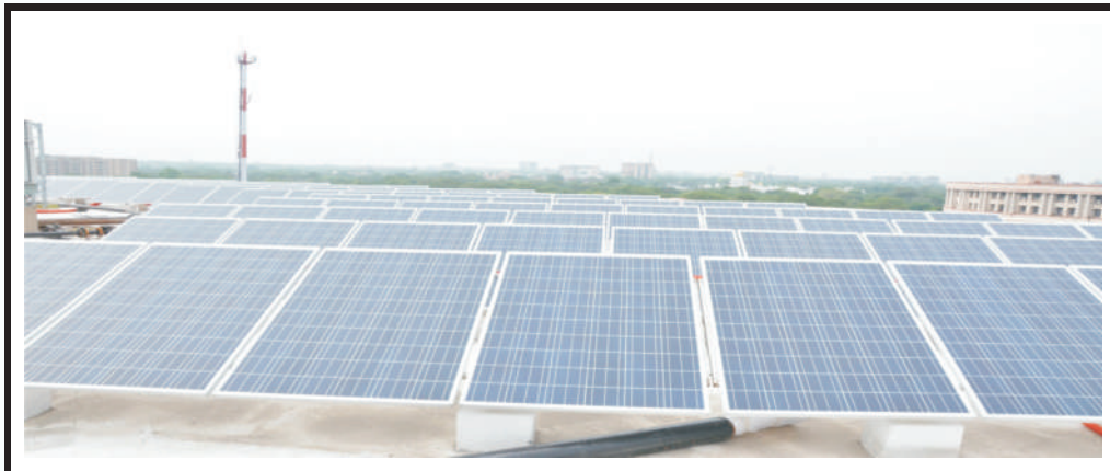
Extension Building to Parliament House Annexe, New Delhi Solar Power - 40KW Peak, saving energy of app. 54,000 units per annum
