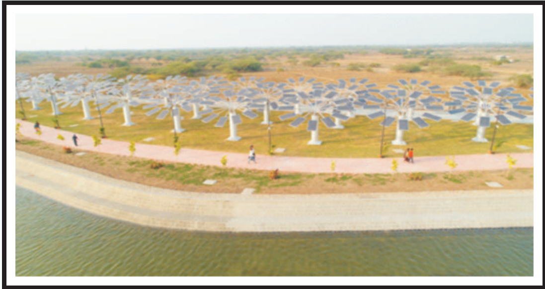
A View of Solar Trees at Dandi Memorial Gujarat
