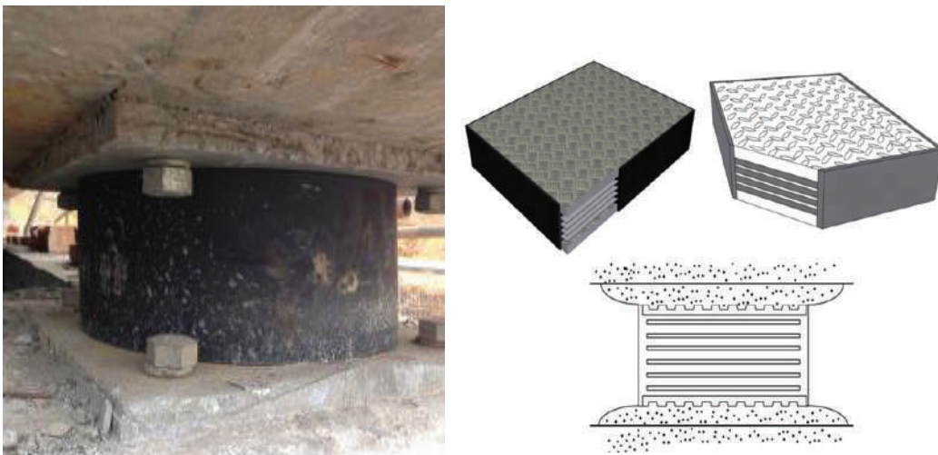
Elastomeric Bearing Pad Laminated bearings with profiled outer steel plates
