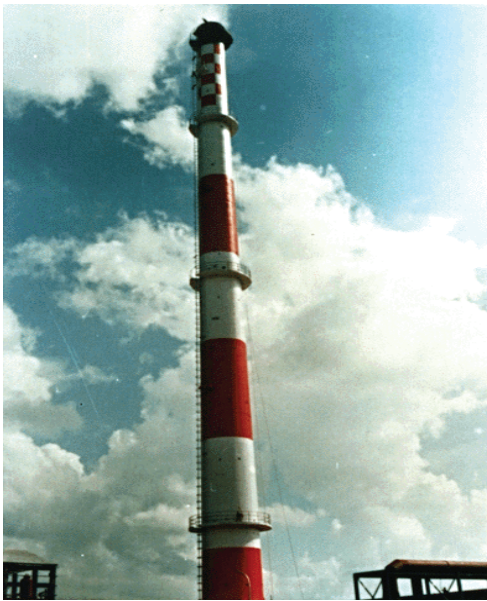
Fig 7: ATV Chimney at Mathura
