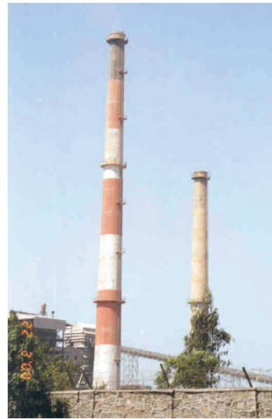
Fig 8: GSEB Chimney at Sika, Gujarat
