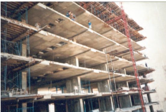
Fig 3: Prestressed Banded Slabs
