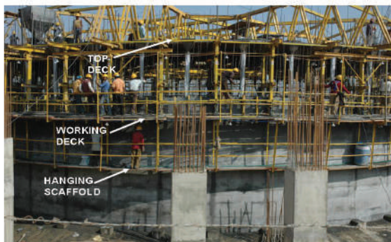
Fig. 13 Slip Forming in Progress
