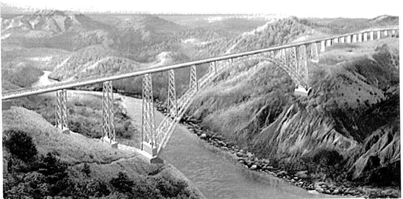
Fig. 30 :Chenab Bridge, J&K (Under Construction), India
