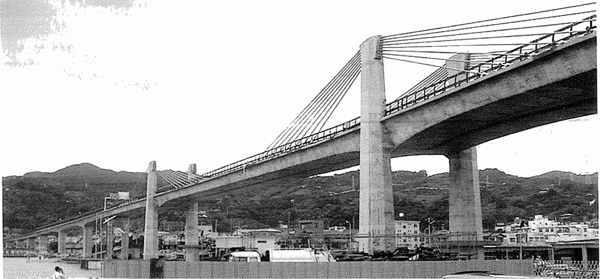
Fig. 16 :First Extradosed Bridge constructed in Japan
