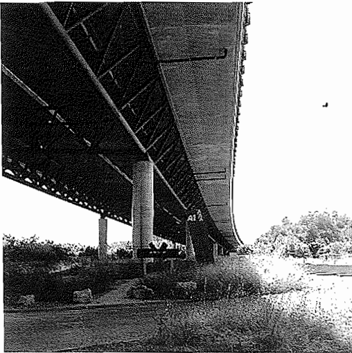
Fig. 23 :The Lully Viaduct, Switzerland
