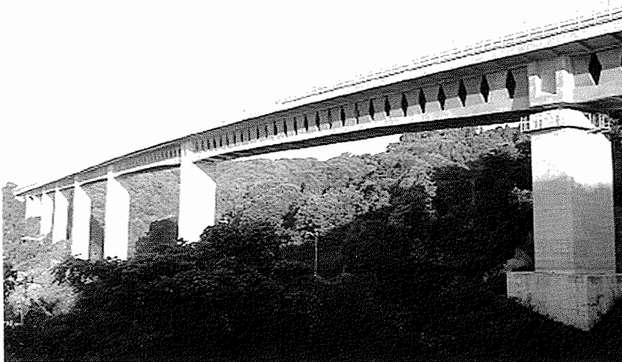
Fig. 21 :Tukubogawa Bridge, Japan
