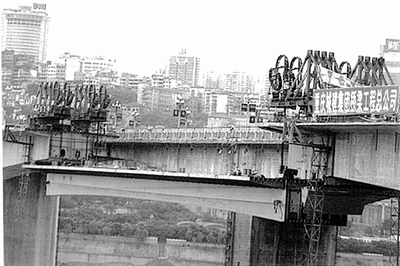
Fig. 18 :Shivanpo Bridge, China Longest Girder Bridge (330m)
