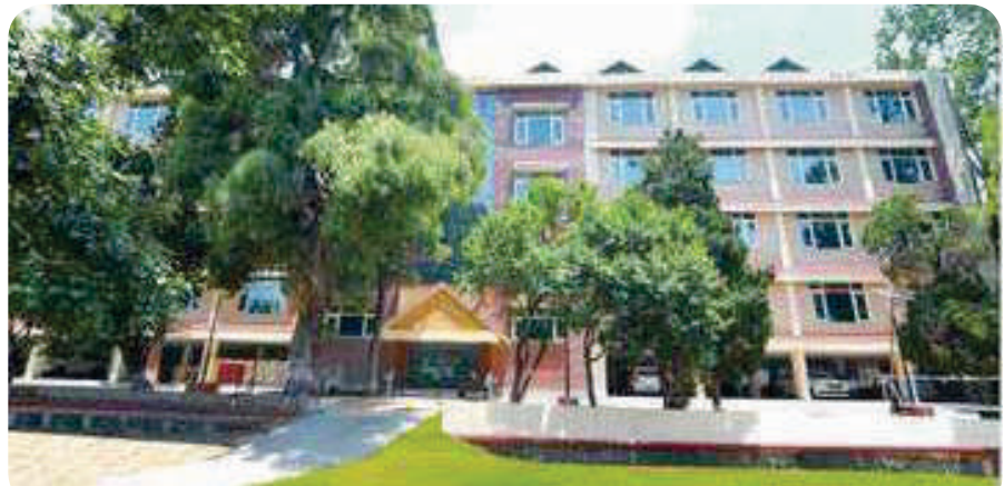
Administrative and training block at SSB TTC, Shimla
