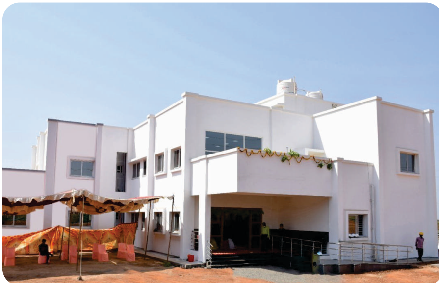
Engineering Block for Indian Institute of Technology, Dharwad
