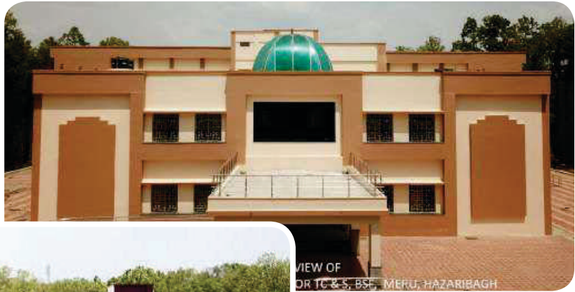
Utility buildings and residential quarters at BSF Campus, Hazaribagh
