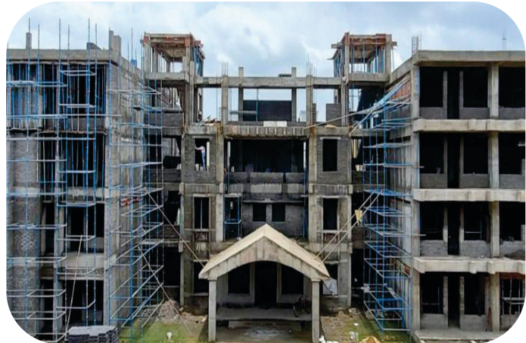
2x180 men barracks for Group Center CRPF at Sambalpur
