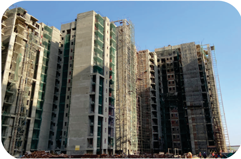
Residential Quarters for CAPFIMS at Maidangarhi, New Delhi
