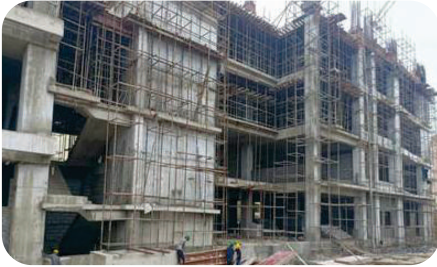
Academic Block and Administrative Block for AIIMS, Raipur
