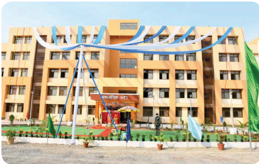
Administrative Building for CRPF at Arang, Raipur
