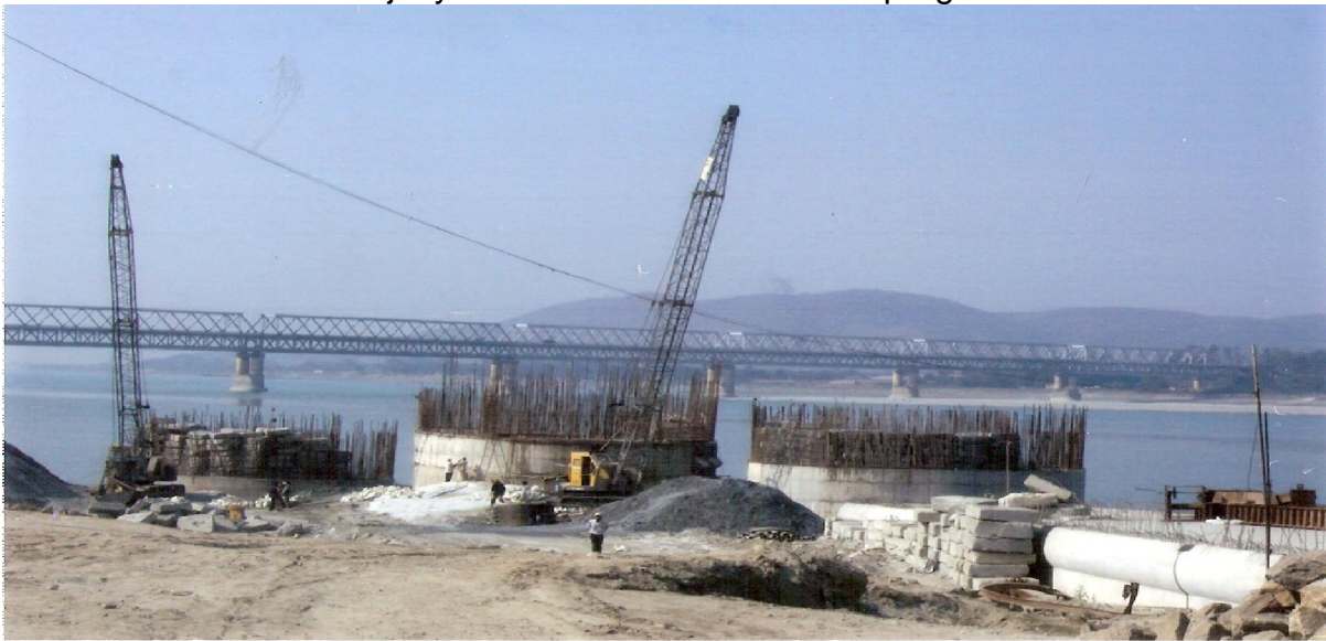
Construction of low level jetty at Pandu, Guwahati
