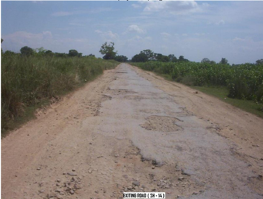
Existing Road Condition
