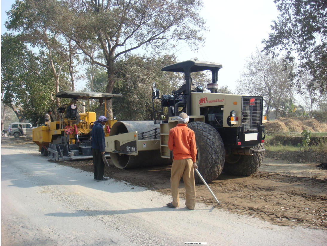
Preparation of subgrade in progress
