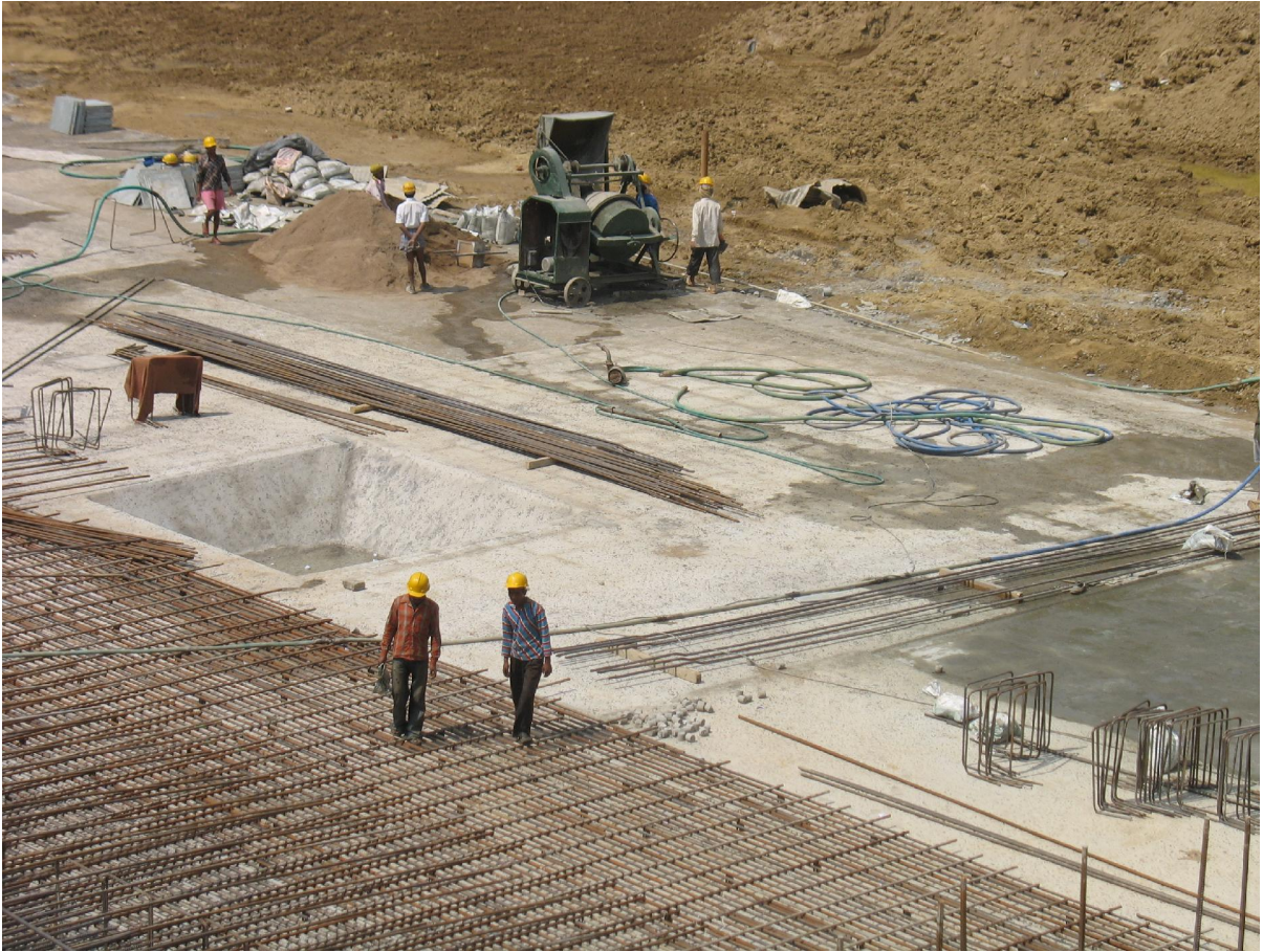
Foundation work in progress at Jawahar Lal Nehru Bhawan
