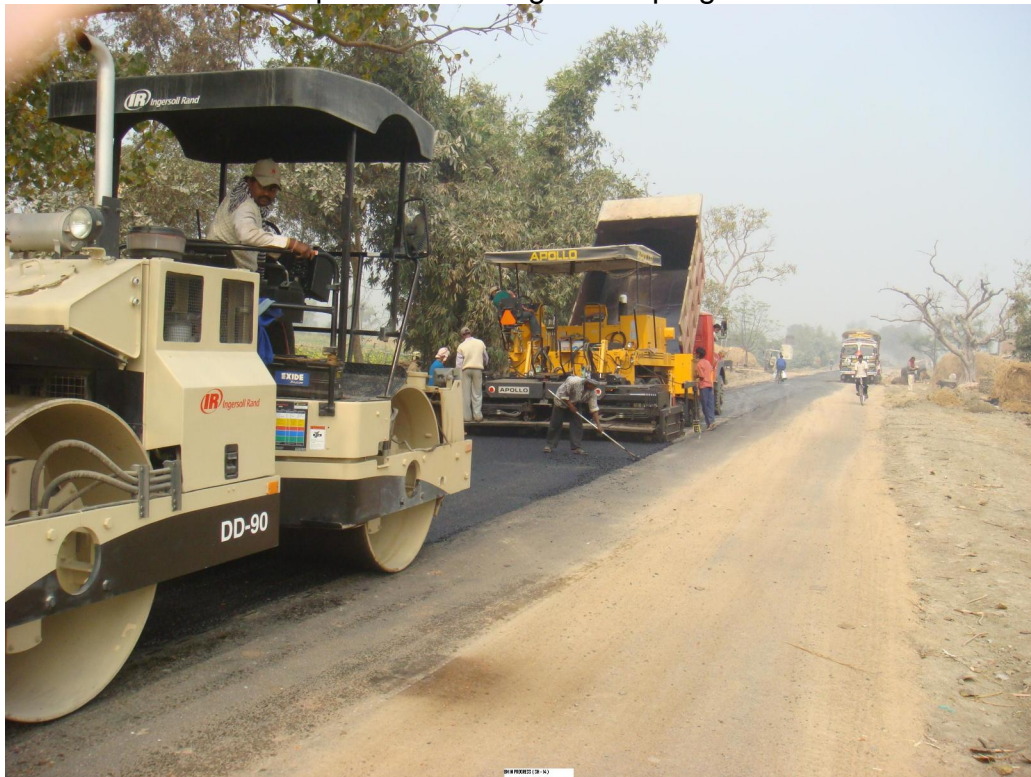
Laying of bituminous surface in progress
